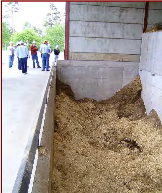
Figure 9: Forest chip bunker, Llungby CHP plant, Sweden
