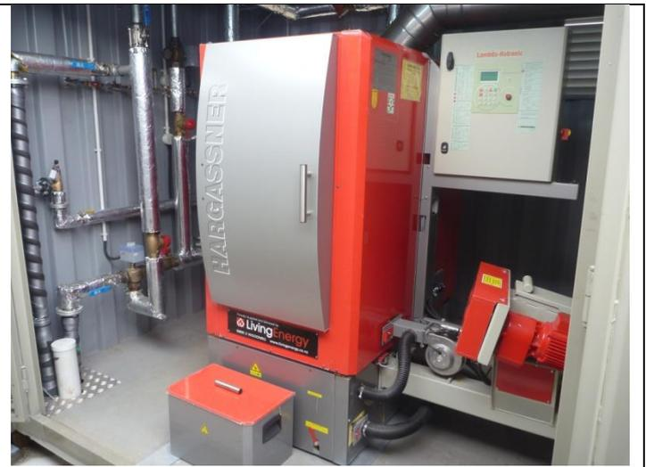
The boiler unit inside the container
