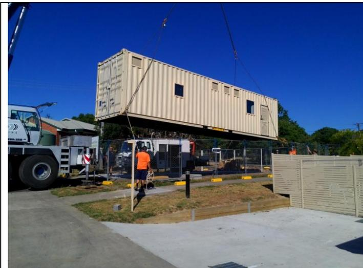
The boiler house being lowered into position
