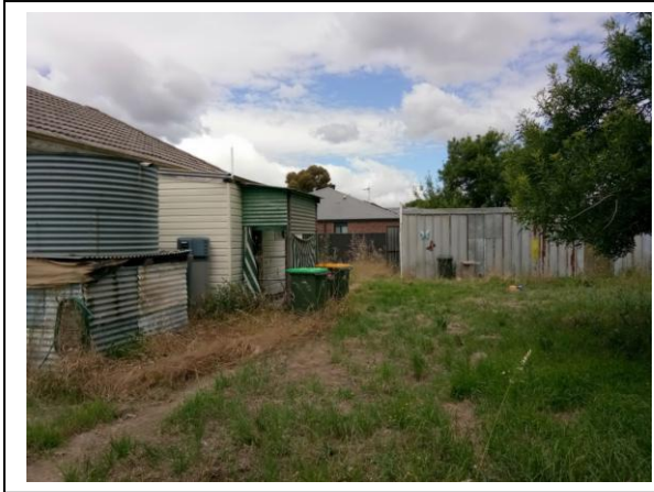
Rear of dwelling with shed to be demolished
