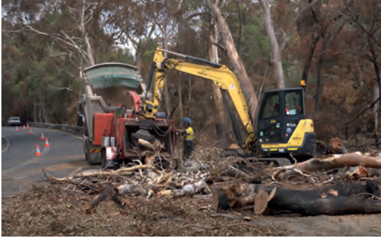
Crews removing hazardous trees in the Main Lead area.
