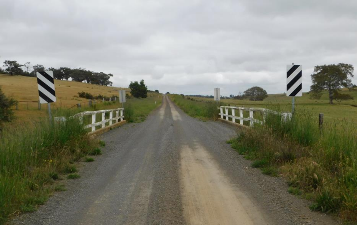
Image 2: Bridge 7 - View from Carngham Trawalla Rd looking west
