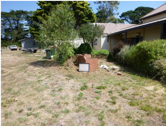
PH16. Approximate location of existing wastewater treatment system servicing residence
