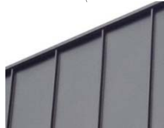
COLORBOND STANDING SEAM CLADDING (COLOUR - NIGHT SKY OR SIMILAR)
