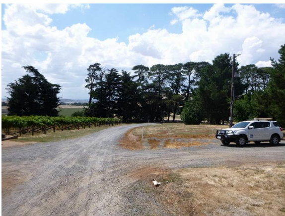
PH36. View over overhead electricity running through northwest portion of subject property
