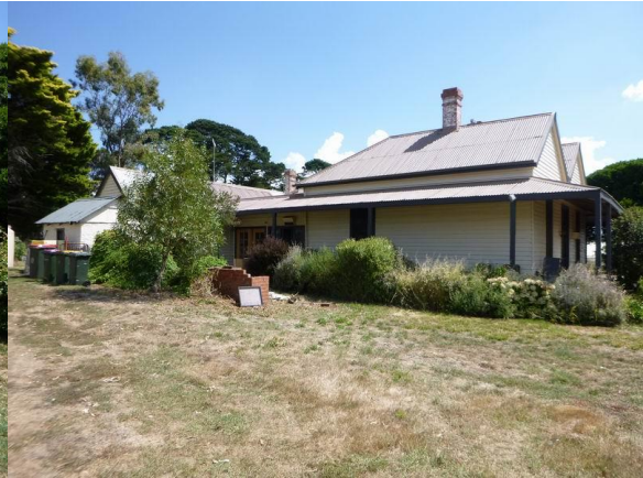
PH15. Existing residence
