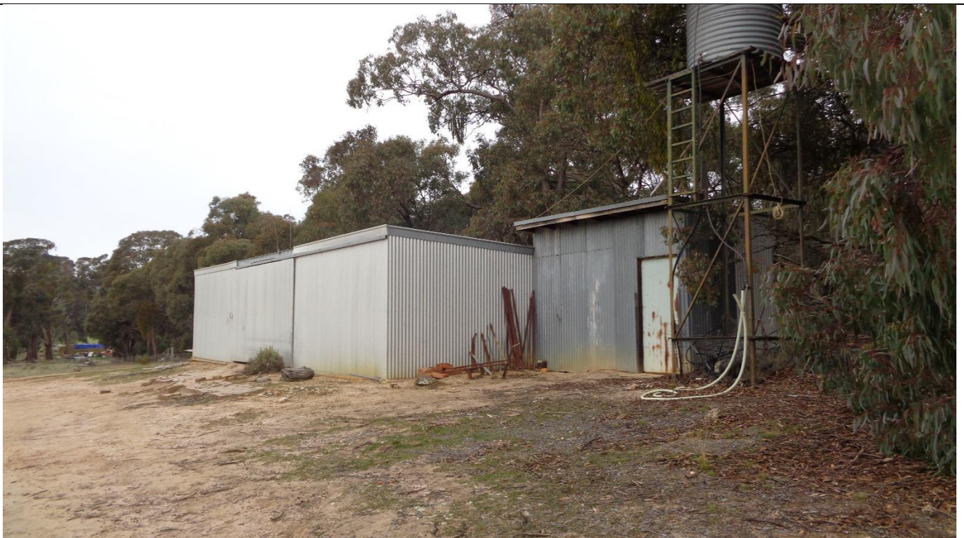
Photo 3 Looking south east to sheds in the south eastern part of the site
