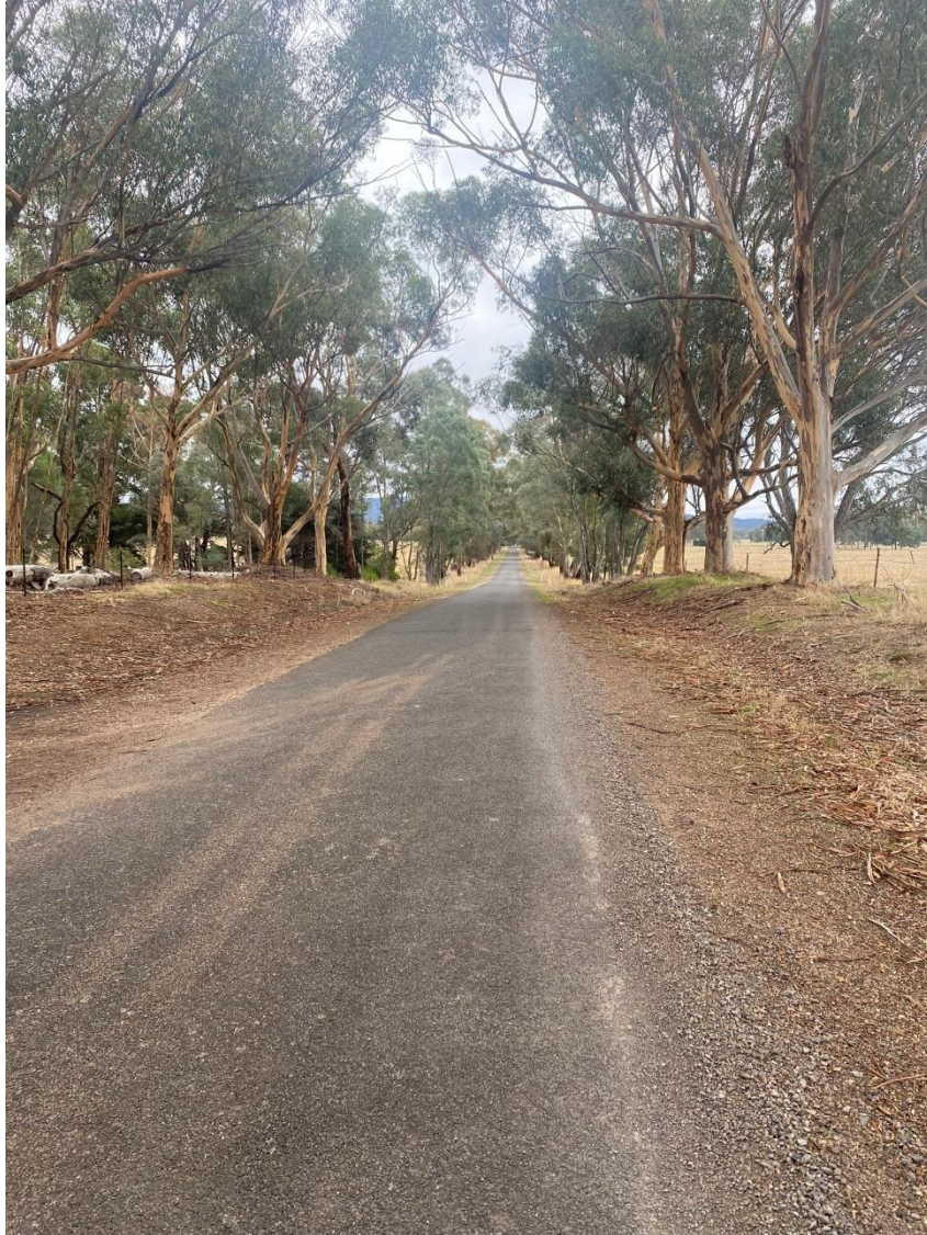
Glenlofty-Warrenmang Road facing east.
