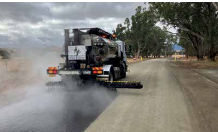
The Crowlands-Eversley Road underwent a $500,000 upgrade this financial year.
