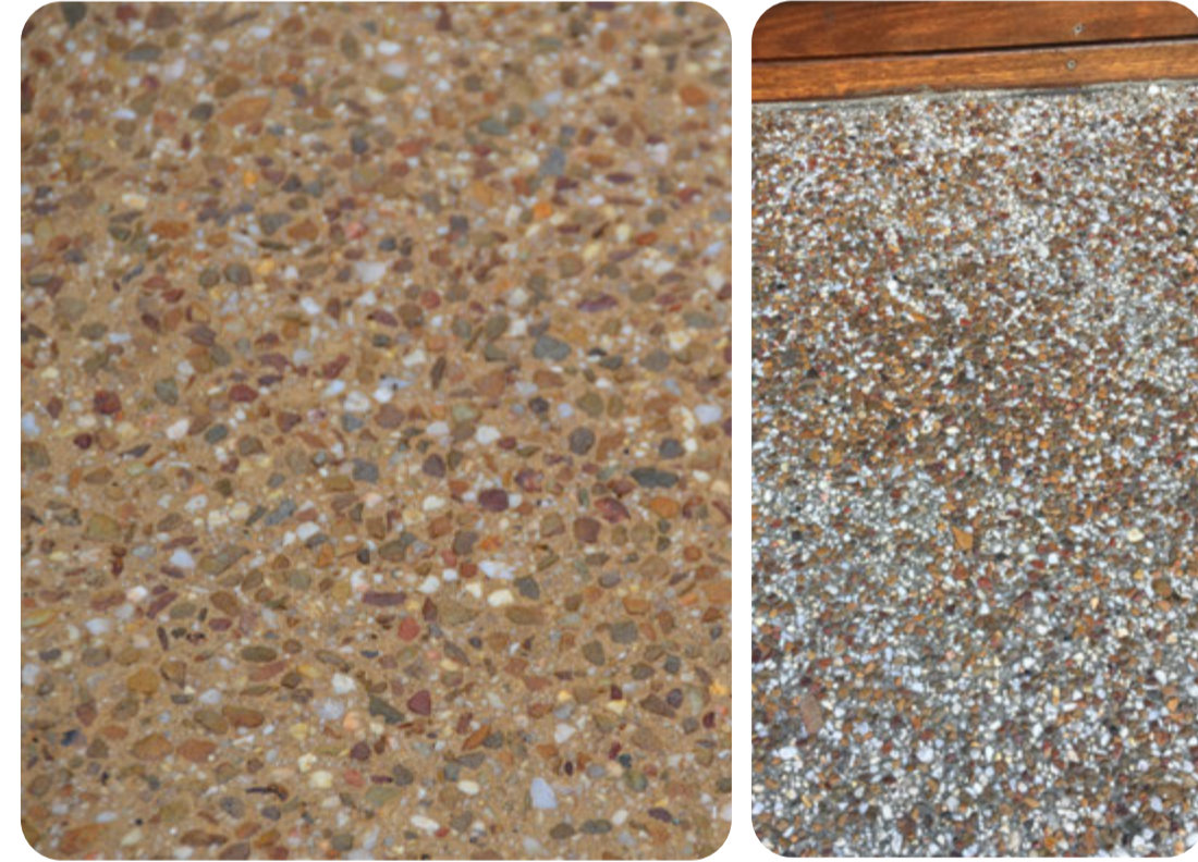
Exposed aggregate concrete paving using aggregates from local Pyrenees quarries
