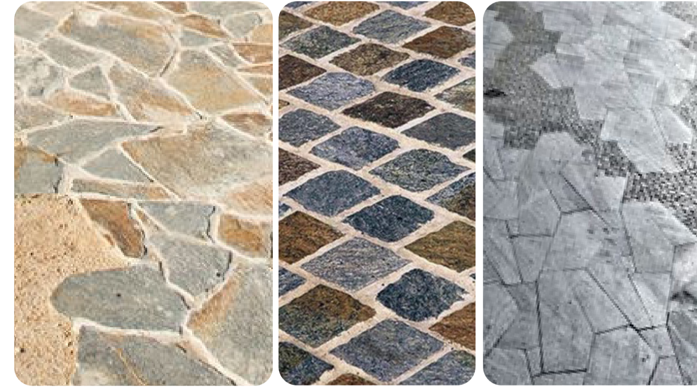
Feature 'River' feature paving along Cambridge Street central spine. Random Castlemaine Slate Stone Pavers/ Cobble Pavers
